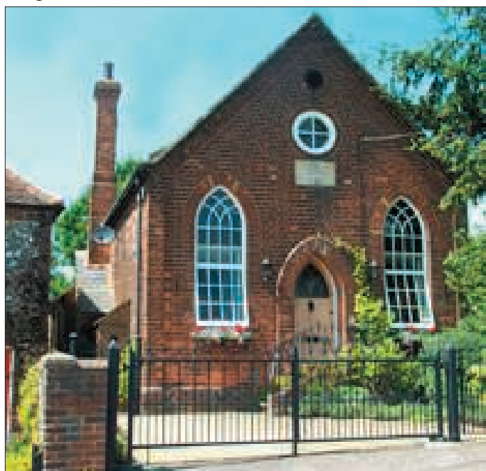
The Methodist Chapel, now a private residence
