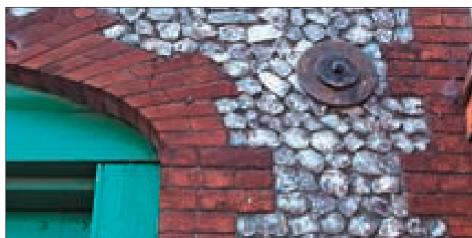
The archway of Flint House, and a detail of the knapped and coursed flint
