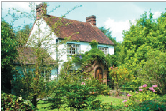
Cherry Tree Cottage, now almost completely engulfed by trees
